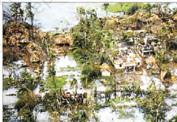
Destruction caused by a cyclone
