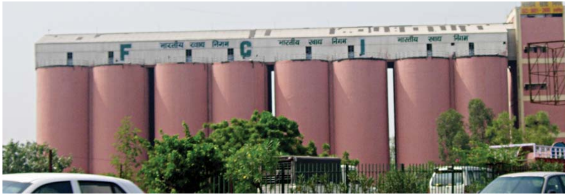
Fig. 1.10 (a) : Silos for storage of grains
